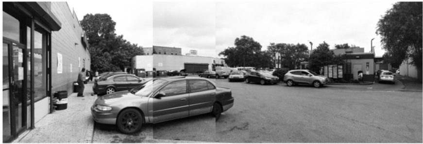
Existing conditions of the abandoned rail right-of-way space where Vernon Walk is proposed. Marginal uses and service functions such as trash storage and drive aisles for drive-thru pick up are scattered throughout.
