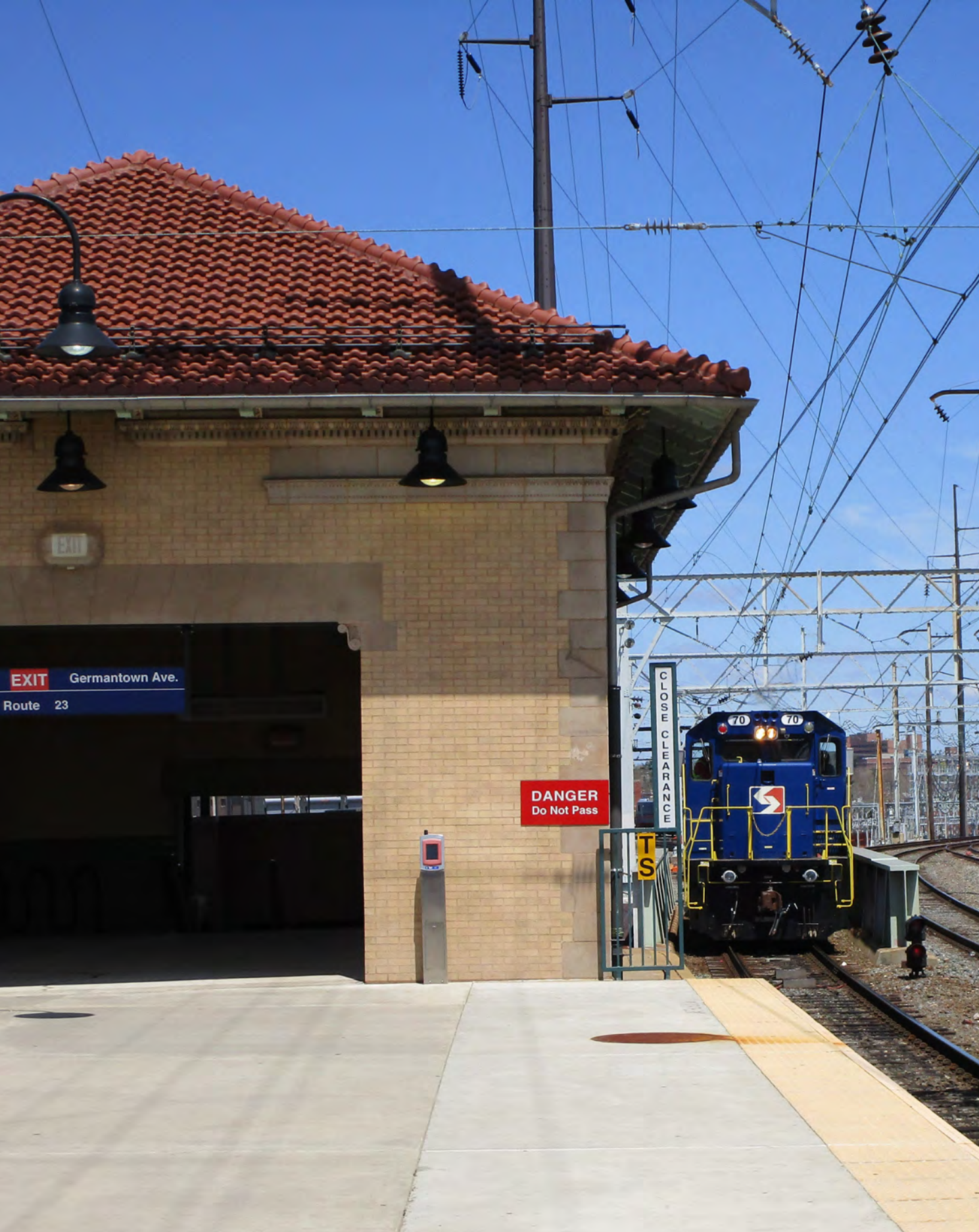
SEPTA completed a major renovation to Wayne Junction Station in 2015.
