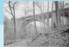
Walnut Lane Bridge Image source: HAER
