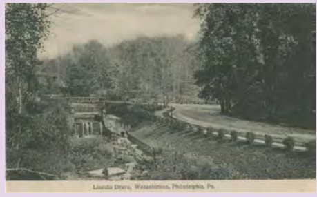
Lincoln Drive with Monoshone Creek on the left, early 1900s. Source: philadelphiaencyclopedia.org
