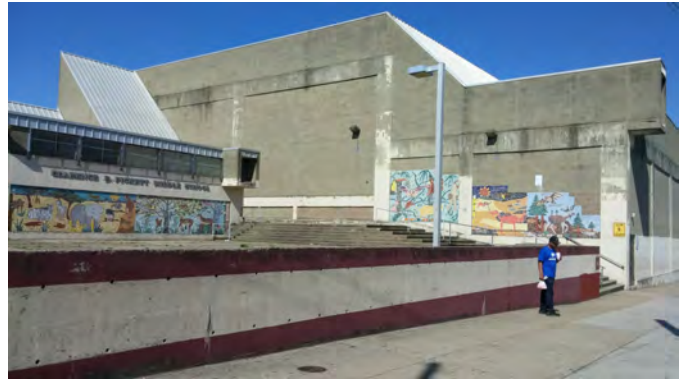
Existing conditions of plaza at Cheltenham and Wayne Avenues.
