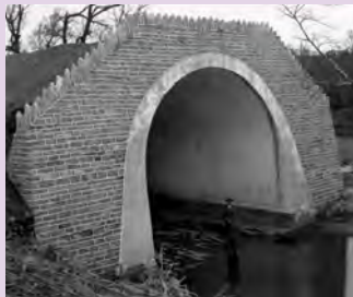
Wingohocking sewer outlet. Source: Department of Records, 1929
