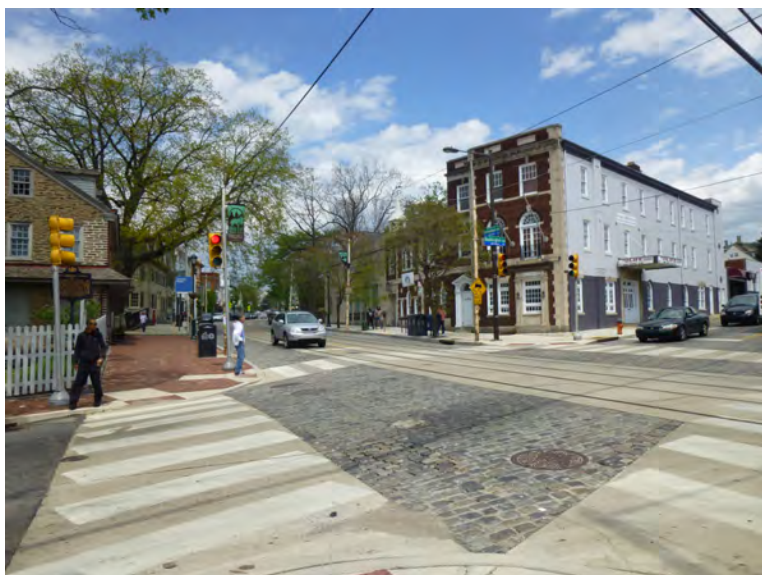
The public realm at Germantown Avenue and Washington Lane is rich with street trees, lighting, overhead trolley wires, banners, building materials, street furnishings, etc. The street materials themselves are historically certified.
