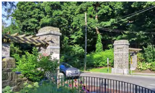
Cresheim Valley Drive pergolas at Germantown Avenue were originally dedicated in 1909 and restored in 2005
