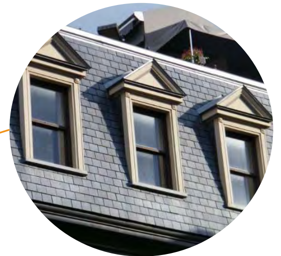
SLATE SHINGLE ROOF
