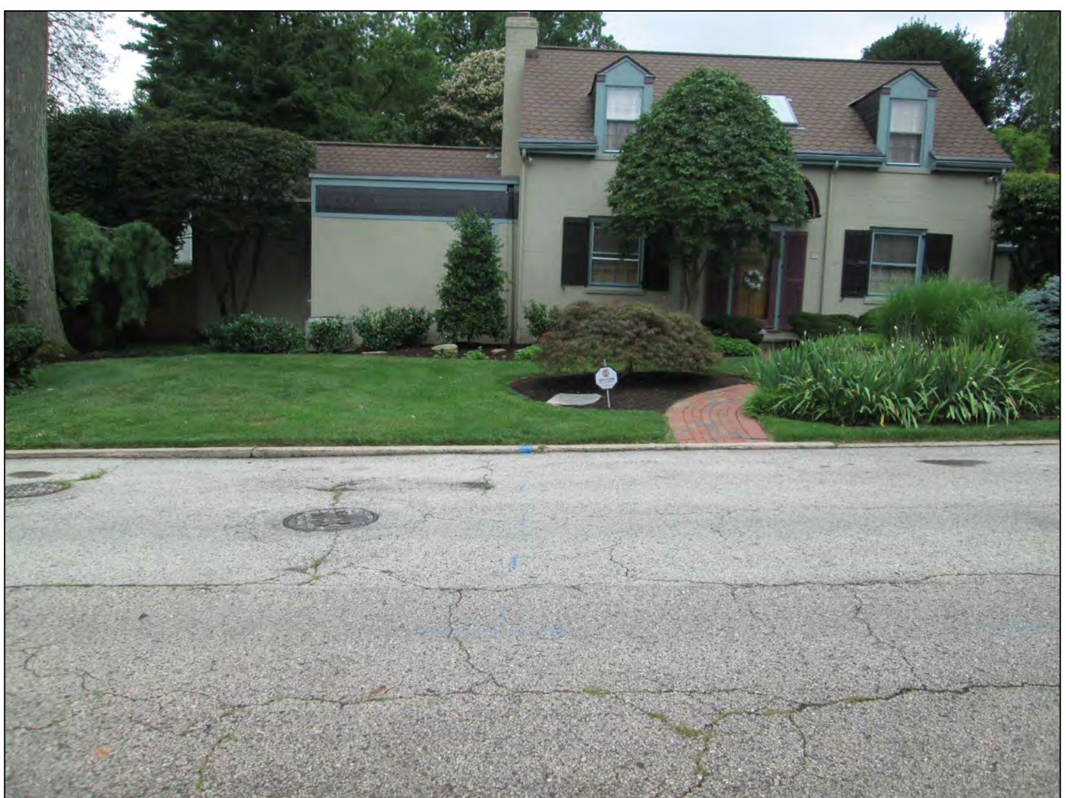
SITE PICTURE OF 101 HILLTOP ROAD "NEIGHBOR TO RIGHT"
