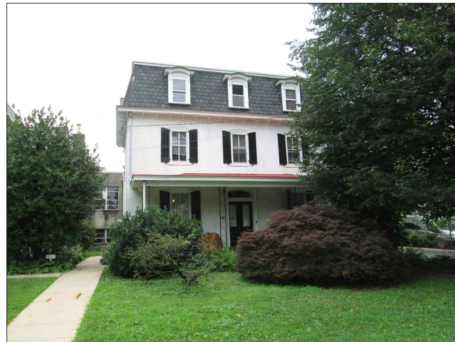
SITE PICTURE OF 8812 GERMANTOWN AVE. SIMILIAR STYLE
